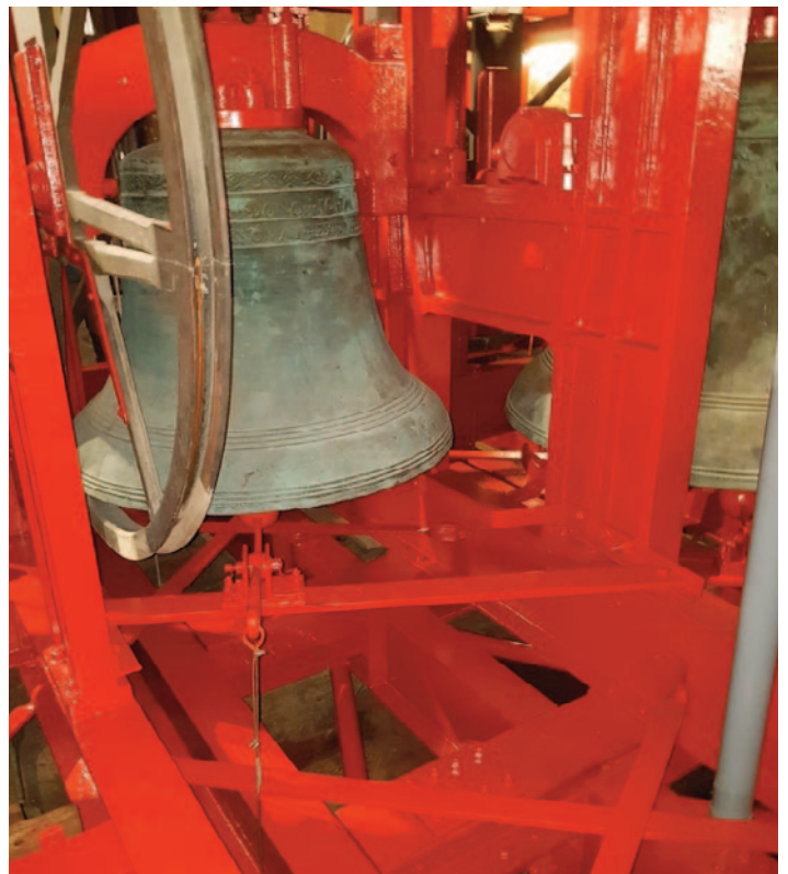
The new strengthening on the base of the frame
