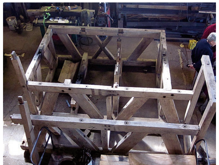
Modifications being made to the wooden frame
