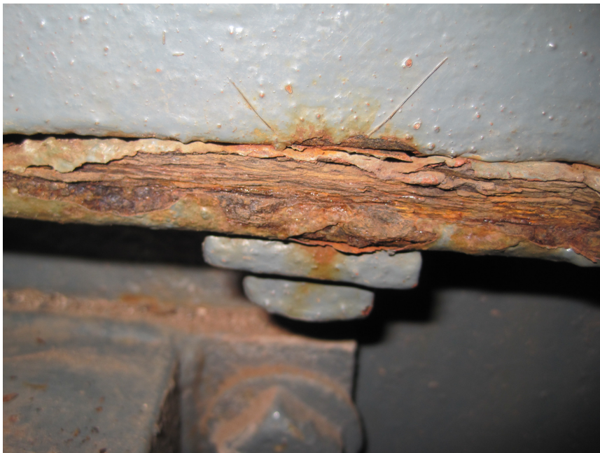
Close-up showing the delaminating of the steel girder
