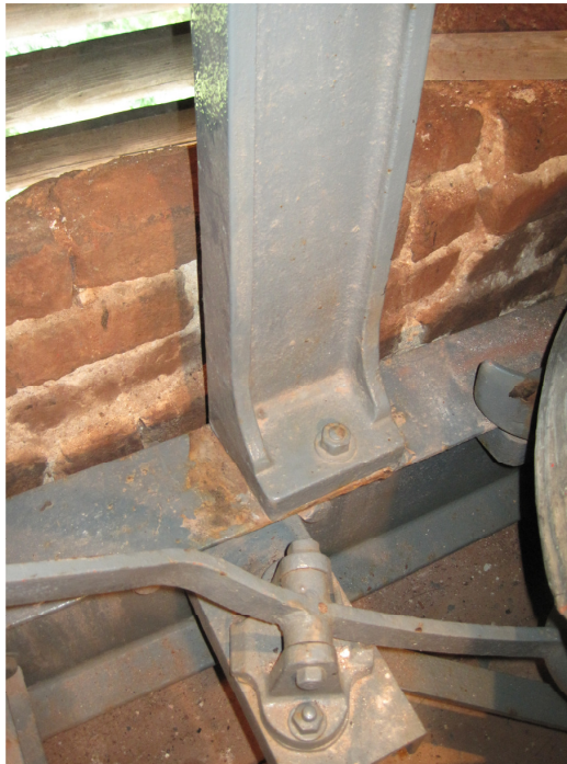
The foot of the H-frame supporting the tenor
