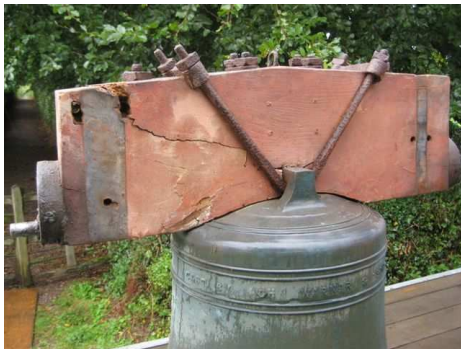
One of the rotten headstocks
