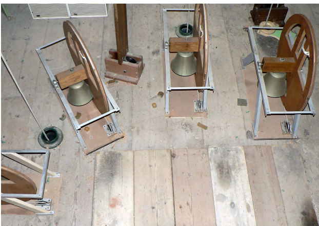
Bells in individual frames in the intermediate chamber
