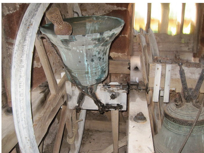
The treble on the left (in the up position) with the second to the right (down). Note the iron band around the top of the second.
