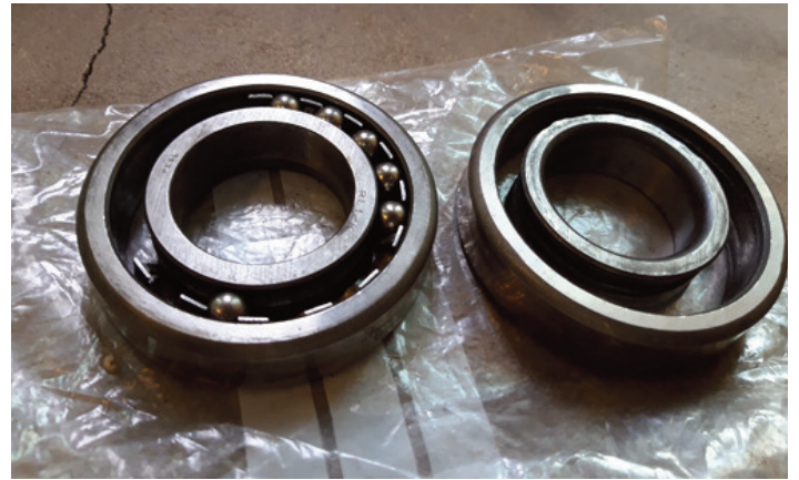
All that was left of the St Mark's bearings
