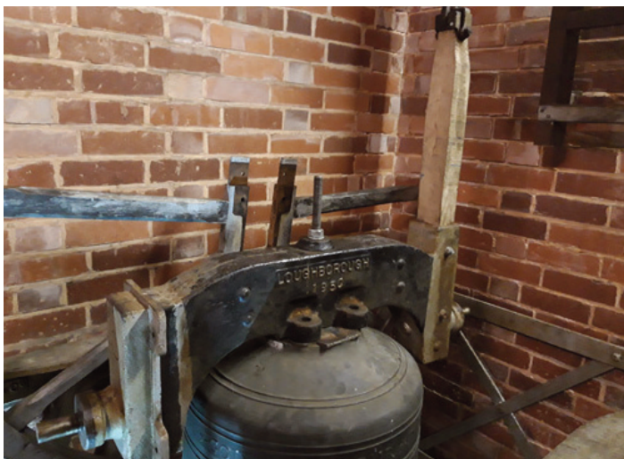
St Mark's 9th with headstock turned 90 degrees and bearings removed
