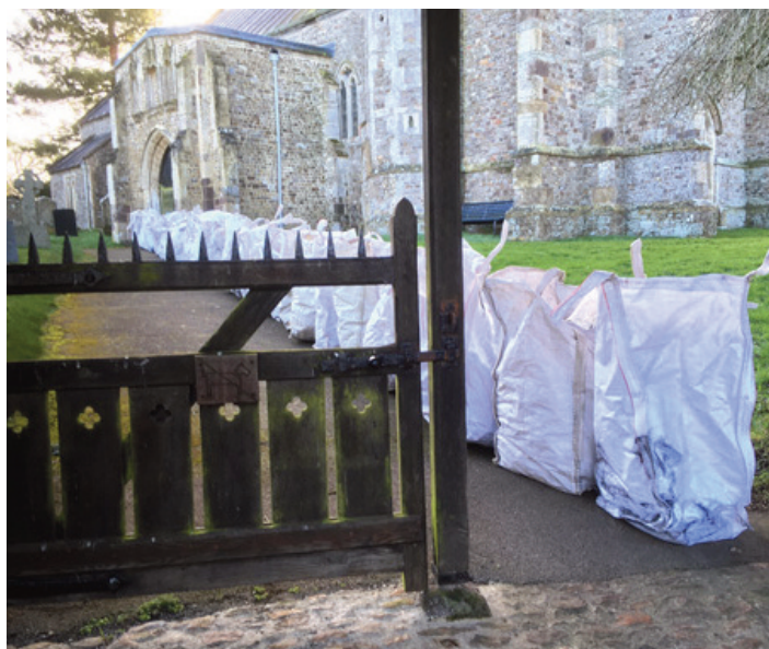
The five cubic metres of jackdaw debris removed from the bell chamber – all bagged up and ready for the compost heap
