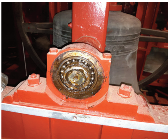
The bearing before being removed
