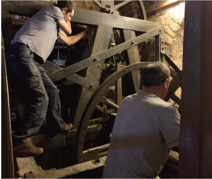
Tower captain Mark Wonnacott and ringer Garry Bater tackle the awkward task of adjusting frame bolts in the tower (©Isabella Whitworth)
