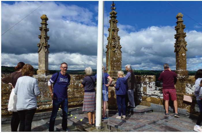
On the tower roof – St Peter's, Tiverton
