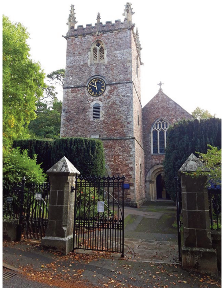
The church at Bishopsteignton
